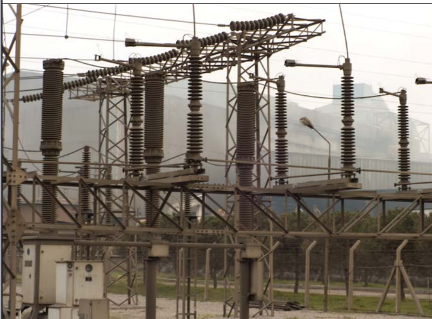
Si-Coat HVIC solved the frequent insulator failure issues from the cocktail of contaminants exhausted at this notoriously polluted steel recycling plant in Western Turkey.
