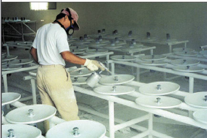
The manual application of Si-COAT HVIC to thousands of insulator discs in 1996 for KAHRAMAA's Phase IV Transmission Expansion Project
